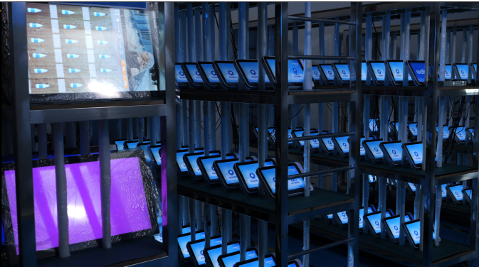
Powered aging room in operation
